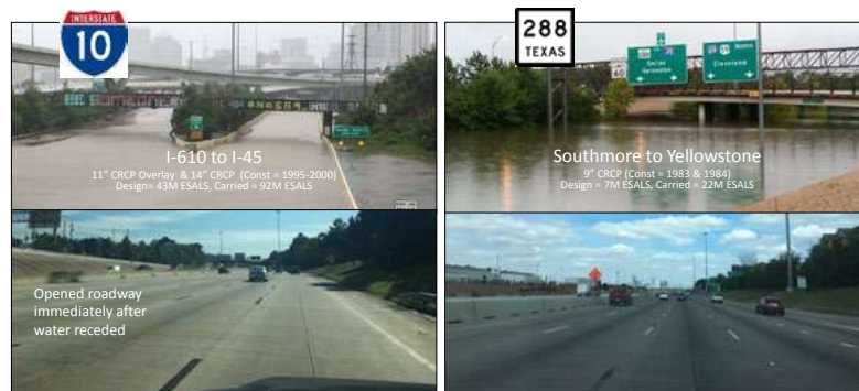
Figure 9: Concrete Pavements in Houston TX. Top shows the roadways when flooded and the bottom shows the open roadways after the water receded
