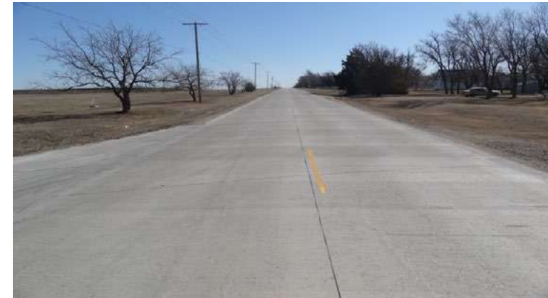
Figure 12. Completed RCC Paving at East 45th Street, Wichita, KS
