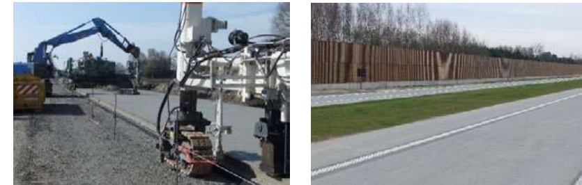
Figure 6. Construction and finished project of the North-South Kempen Link, Geel-Kasterlee, 2013
