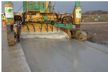
Figure 2. Laying of the white top layer titanium dioxide of the two-layer pavement in Wijnegem
