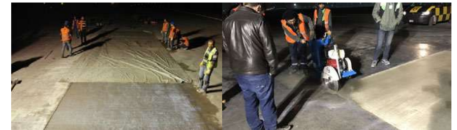
7. Concrete curing
