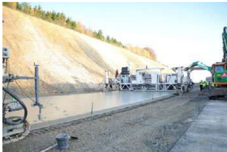
Figure 8. Construction of the 2nd phase of the Couvin bypass (photos @ Cimbéton)
