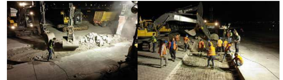
1. Breaking and removing the old slabs
