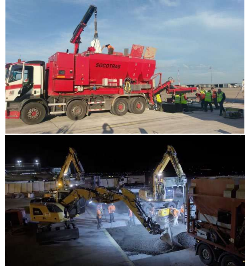
Figure 9. Mobile batching plant and night time renewal.
