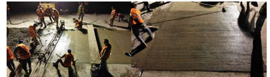
5. Concrete compaction and vibration
