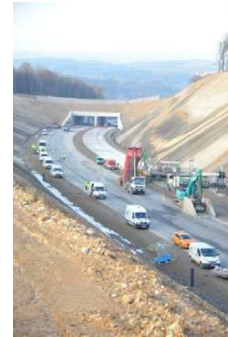
Figure 9. Concreting over the entire width with two slipform pavers (photos @ Cimbéton)
