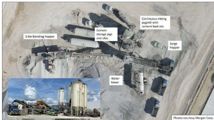
Figure 6: Aerial and elevation views of continuous pugmill mixing operation for large-sized RCC paving projects
