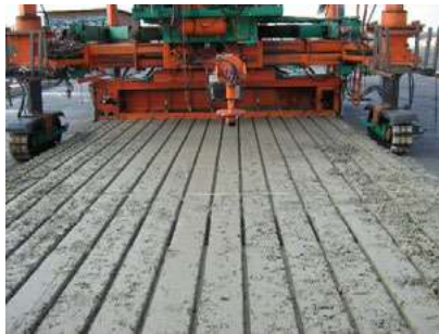
Figure 11. Lommel Kristalpark - placing dowels in the slots in the bottom layer
