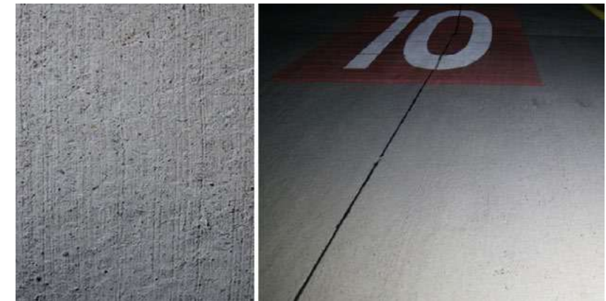
Figure 4. Photo of the slab repaired in 2004 after 11 years (2015).
