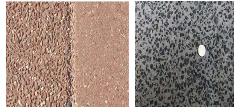
Figure 1. Exposed aggregate concrete surfaces – homogeneous and contrasting combination of stones and mortar
