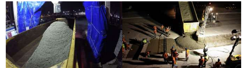
3. Concrete production at the plant
