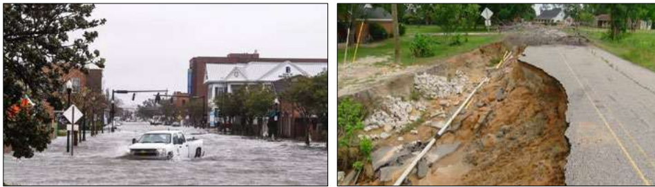
(a) Pavement Inundation (left) and Washout (right) Impacts
