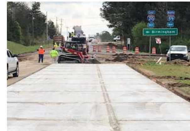
Figure 13. Installation of RCC Paving at McAshan Road in Bessemer, AL
