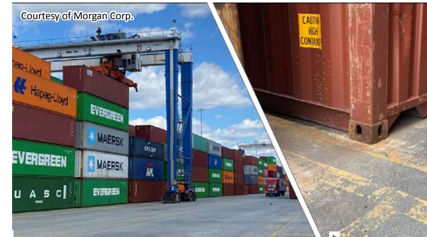
Figure 2: (a) General view of RCC pavement at a container handling facility, and (b) a close-up view of a container corner casting bearing on RCC pavement
