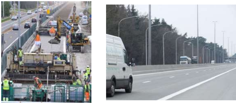
Figure 5. Construction and finished project of the E213, Herentals, 2012
